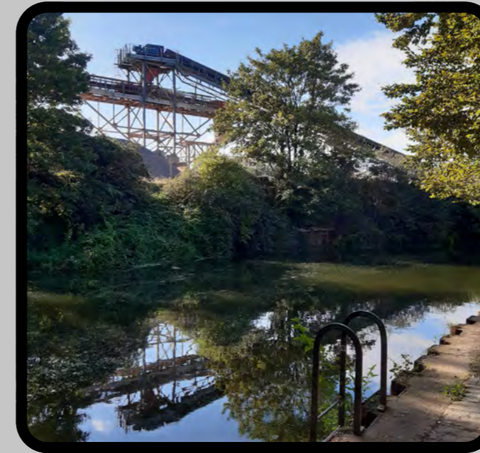
...and used to construct roads, homes, schools, hospitals and other buildings
