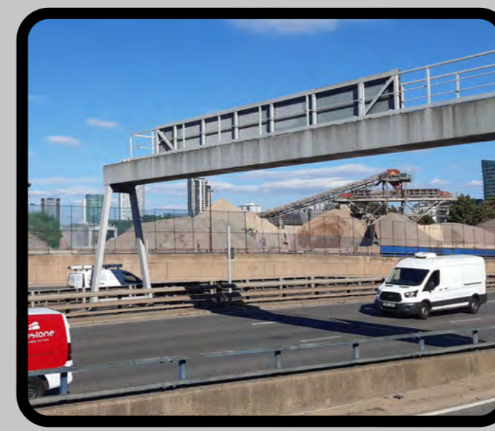
These are moved in and out of the site by rail...
